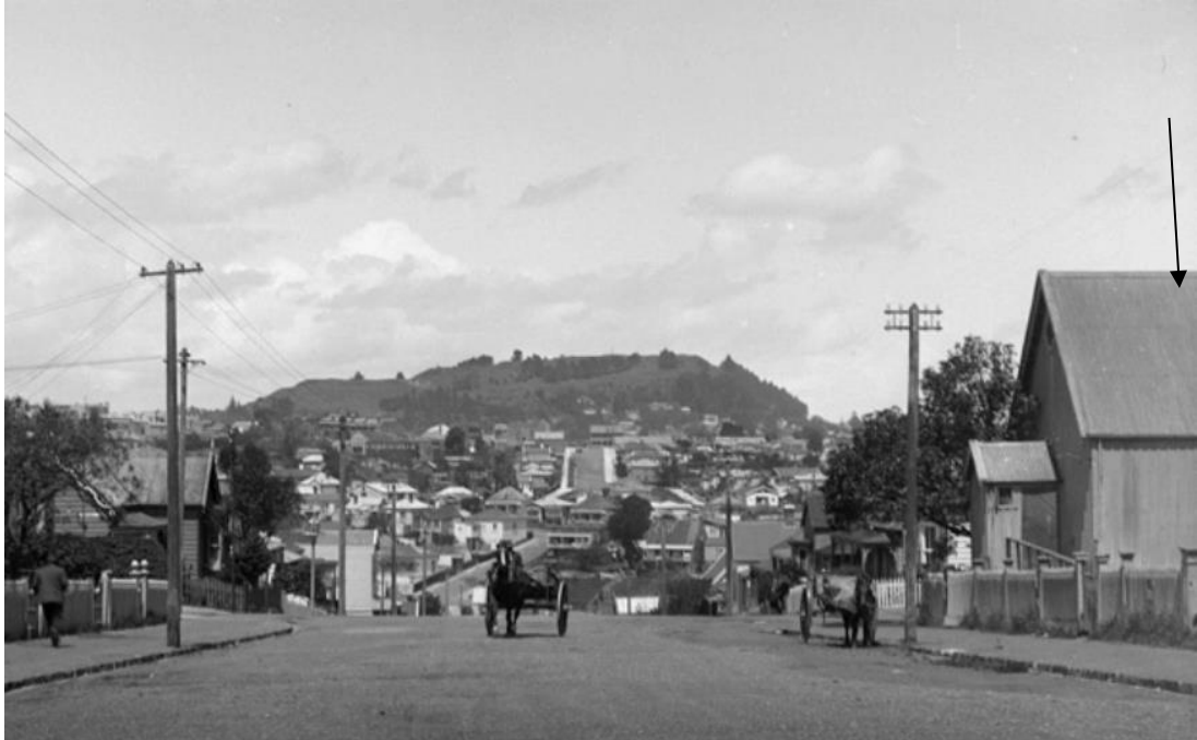
Figure 14. Photograph looking south down Gundry Street dated 1924 with the Church Hall indicated by the arrow (source: Digitalnz.org/records/30079540)
